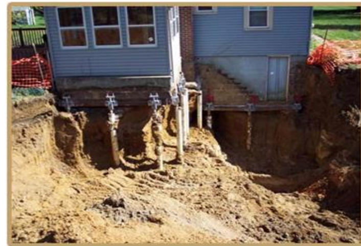
Sequence of the helical pile underpinning of existing foundations (Lutenegger & Kemper, 2008) and performing helical piles
